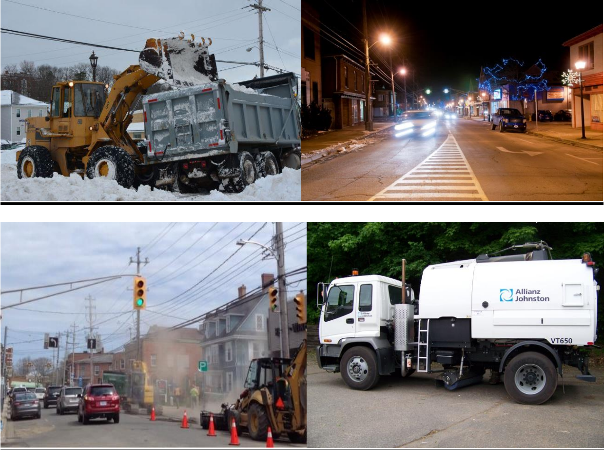
Clockwise from top left: Snow removal after storm, street lighting, street cleaning equipment, paving.
